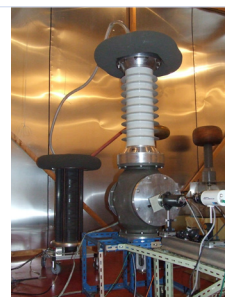
Cellule HVDC 350 kV
